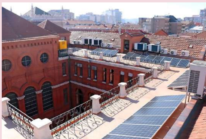
Image 2. Installation of solar panels on the roofs of municipal buildings
